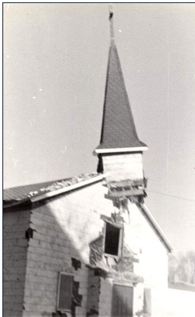
The barracks chapel goes down to make room for the building of the new church.
